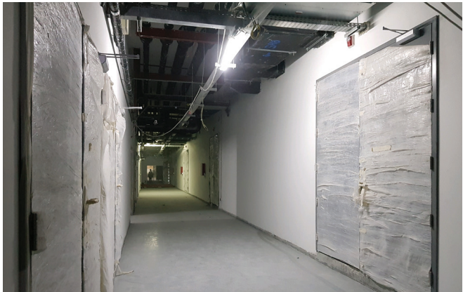
Completion of fire rated door fixing in the basement, LR, UR area
