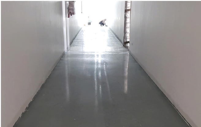
Epoxy paint work in the corridor of lower retail
