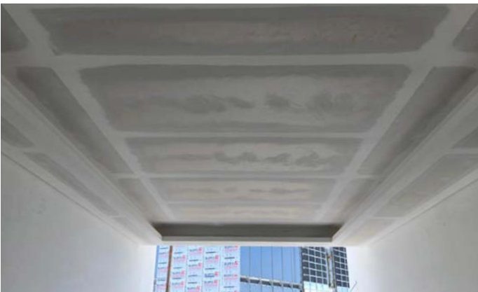
Gypsum ceiling in progress
