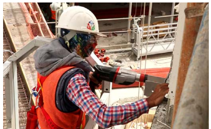
Fixing of extract fan - Upper retail level
