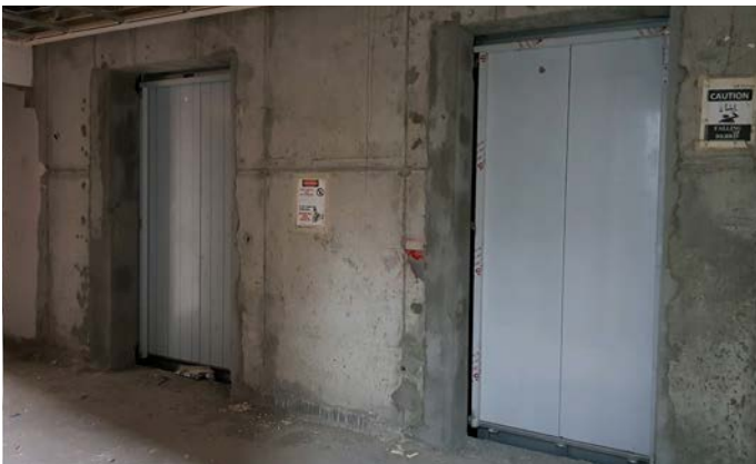
Completion of lifts door fixing - Typical floors
