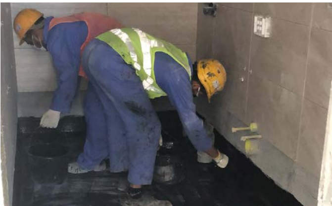
Water proofing works in the wet area
