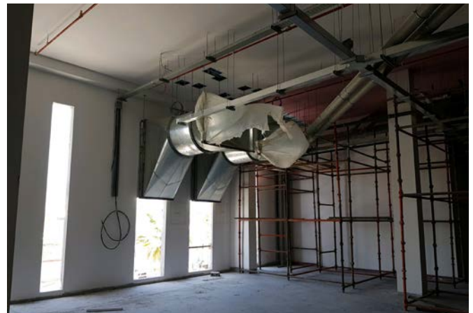
Fixing of extract fan - Upper retail level
