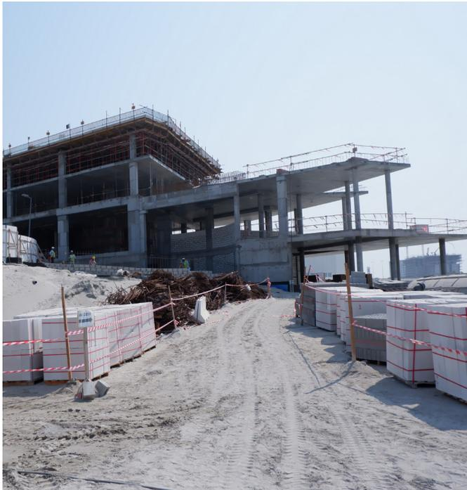
Shuttering, Reinforcement and Concreting of amenity floor slab in progress (30% complete)
