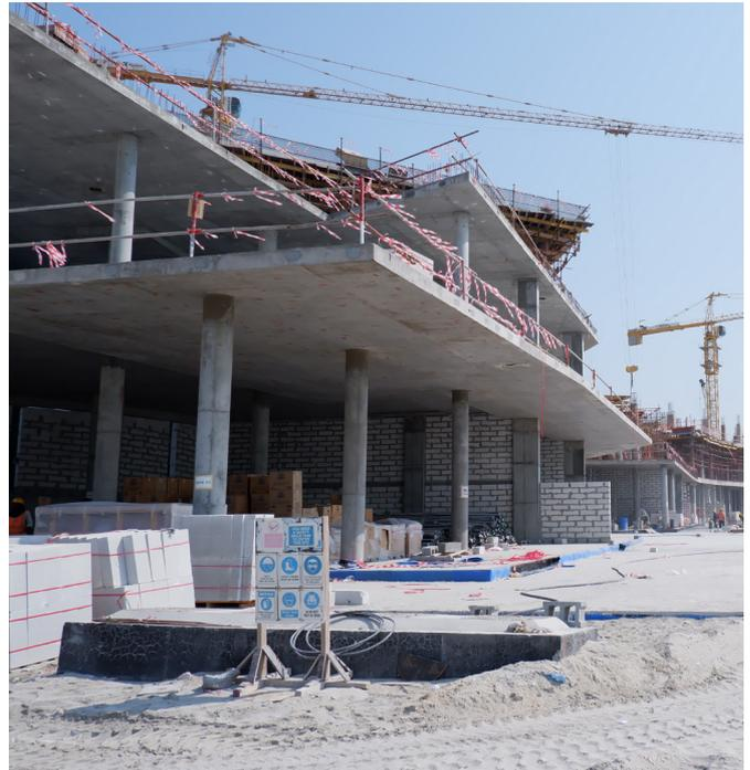
Column Shuttering, Reinforcement and Concreting of initial Amenity level residential block A floor in progress (15% complete)
